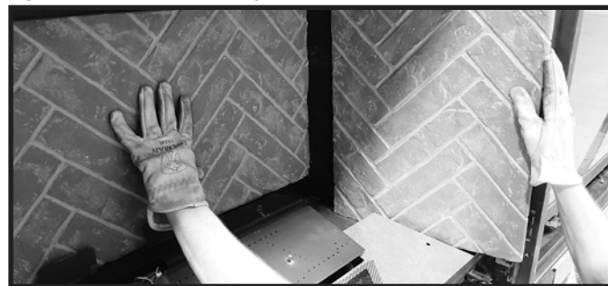
Figure 11.3 Install Side Refractory Panel (Right Side Shown)
